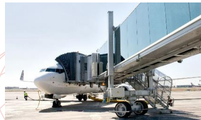
Passenger Boarding Bridges
